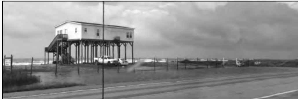
Last house traveling east before the curve, June 29, 2017, picture by Pam Reber
