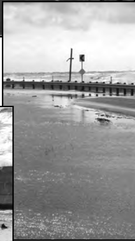
Guardrail at Hwy 87 and Hwy 124 curve fallen barricades in background. Pictures by Pam Reber, June 29, 2017
