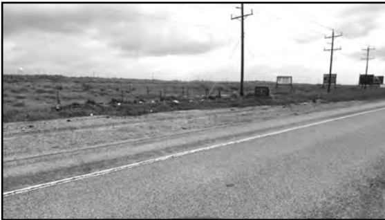
Sand washed over highway filling drainage ditches June 29, 2017, picture by Pam Reber
